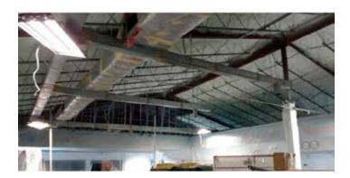
A complex maze of service catwalks needed for old HVAC equipment is removed as part of each building's renovation process, exposing ample room for new Daikin equipment.
