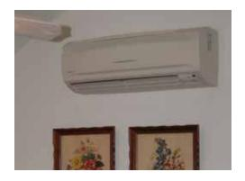
Aslan proposed using three 2-ton multisplit Daikin MXS heat pump systems, a simpler and more cost-effective multi-zone solution that fit the mansion perfectly. These replaced the two ailing 5-ton single split systems for a 40% reduction in tonnage that would take full advantage of building diversity and translate into good energy savings.
