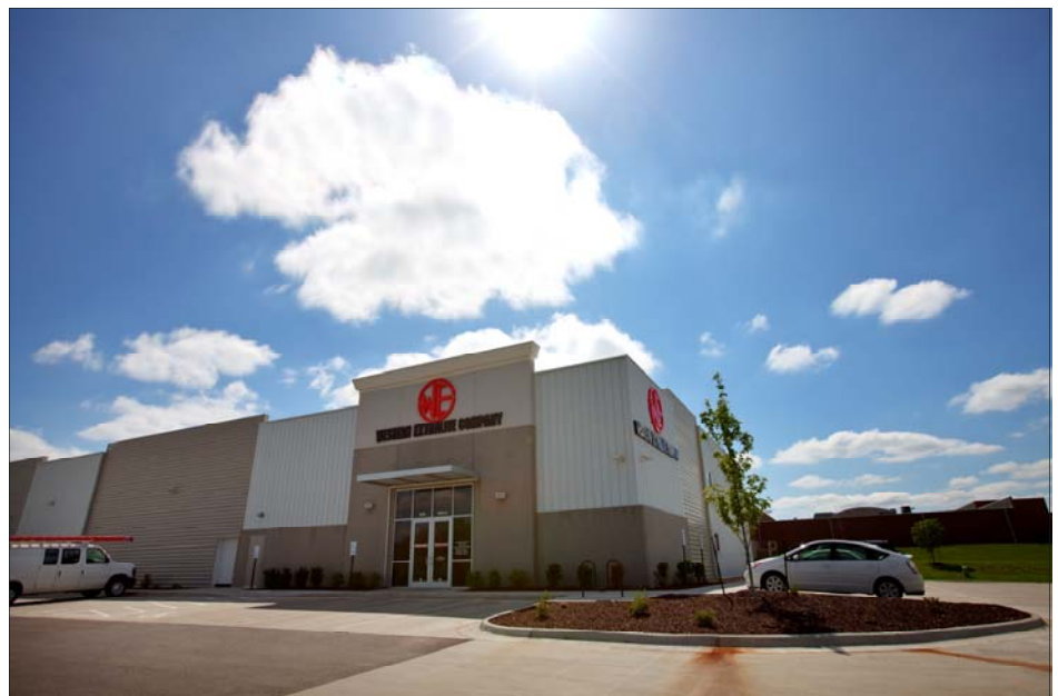
The Daikin system installed in Western Extralite’s Lawrence facility was named the city’s first LEED certified private business, and was awarded LEED Silver certification in January 2010. Owners cite the energy consumption of the 20,000-square-foot space is similar to the energy used in their old 12,000-square-foot building.
