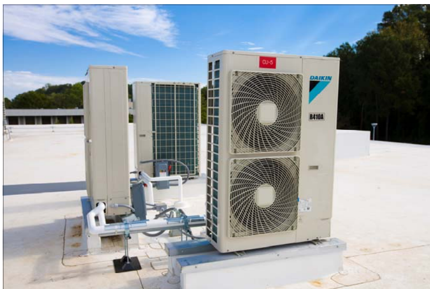
The HVAC system included a Daikin VRV ® -S Heat Pump System. Design and installation of the inverter-controlled systems was supported and serviced by Daikin during the project.
