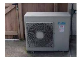
Daikin 4MXS32 and 3MXS24 outdoor units were used to supply the slim ducted indoor units, which now served seven individual comfort zones. The homeowner used the standard wireless remote controls, and especially enjoys the "Dry Mode" feature. This helps reduce humidity in the home during the shoulder seasons with maximum efficiency and improved comfort.
