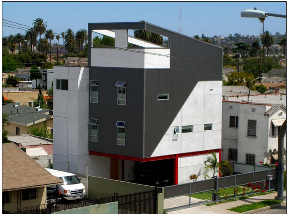
The 1,600-sq.-ft. home in Los Angeles designed and built by architect Jayna Cooper is a model of sustainability. It includes an energy-efficient, duct-free Daikin AC® 4-port Multi-Split system for heating and cooling.
