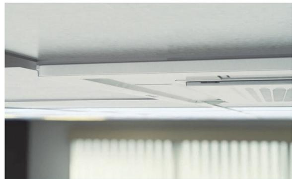
The VISTA™ decoration panel depth measures a mere 5/16" (8 mm), discreetly blending with the ceiling face.
